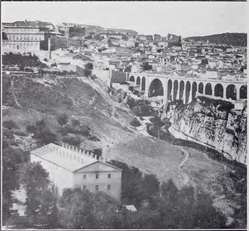
No view in North Africa is more impressive bridge spans the chasm which forms a natural fortress and was one of the last Berber cities
